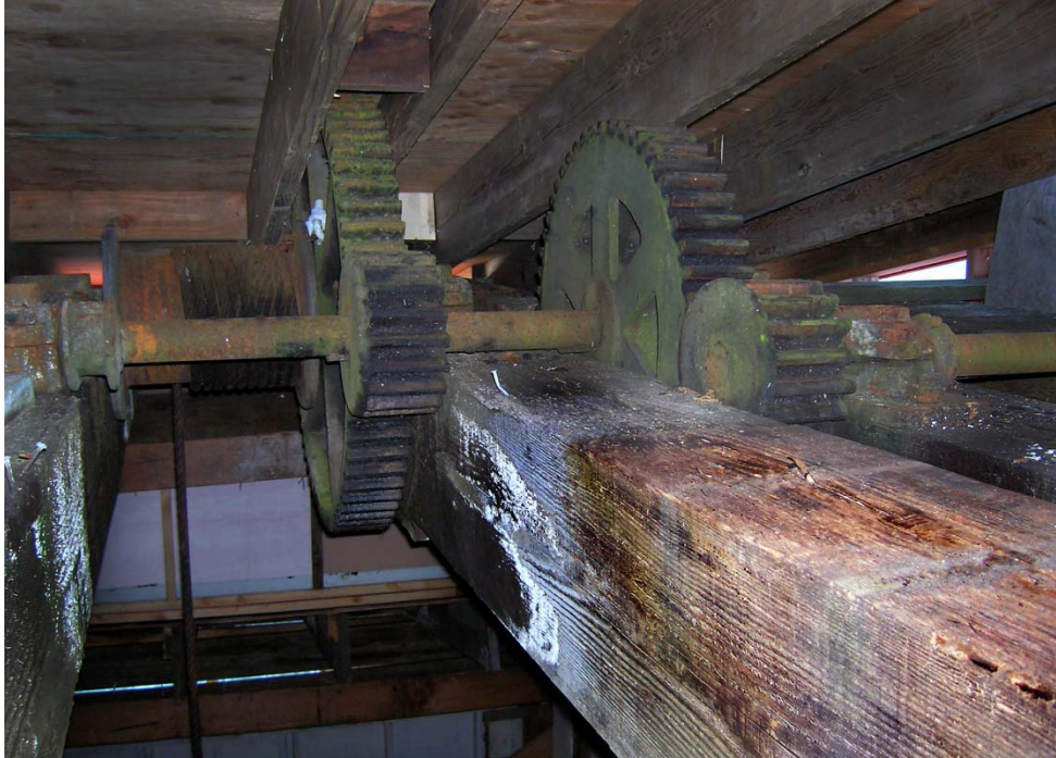
Existing old boat-hoisting mechanism
